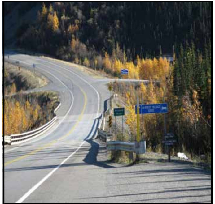
The Triple Lakes Trail parking area at right, the Nenana River bridge and entrances to Grizzly Bear Resort (right) and McKinley Village (left). This area has many safety concerns for both vehicular and pedestrian traffic.
