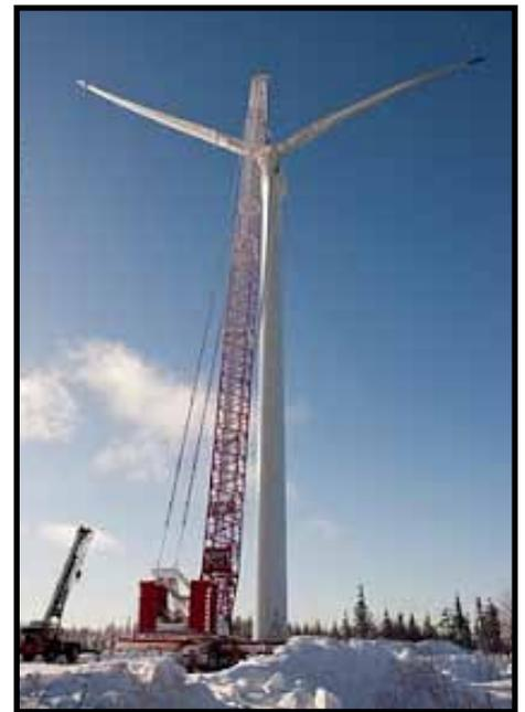
REpower Cold Climate MM92 wind turbine being installed at a site in Riviere-au-Renard, Quebec, Canada. Twelve of these turbines will be installed at Eva Creek.
