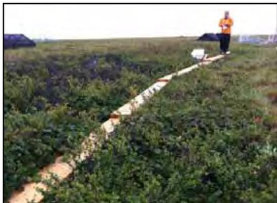
DCC joined Friends of Stampede in preferring a boardwalk-style access path (shown at the Toolik Field Station, above) over the use of Geoblock.
