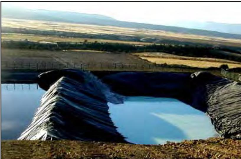
Photo depicts surface storage of waste water at a drilling site in a lined pit. The regulations under consideration by AOGCC do not currently cover disposal and containment of waste water. *photo property of Friends of Mat-Su*
