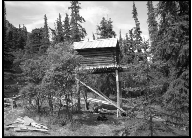
Pearson cache - one of the many historic buildings the Special Projects crew will restore. Photo courtesy of Jean Balay
