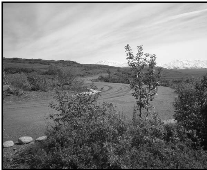
Park road between Eielson and Wonder Lake, where an extensive rehab project is planned along 13 miles. DCC Photo
